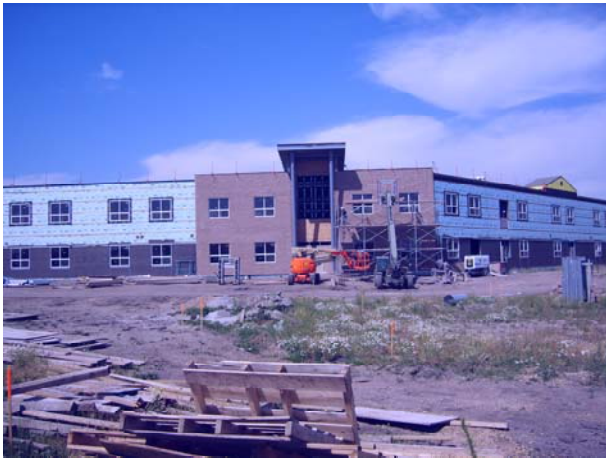
FRONT VIEW FEATURING THE MAIN ENTRANCE
