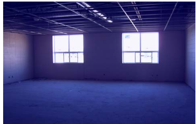
SOME CLASSROOMS ARE ALMOST READY
